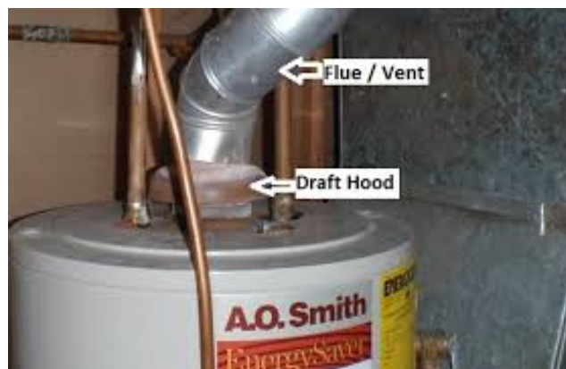
Properly Installed Draft Hood & Pipe
