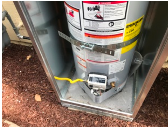
Unsafe Installation of Water Heater Gas Line
